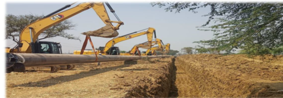
Setting up slurry pipeline
