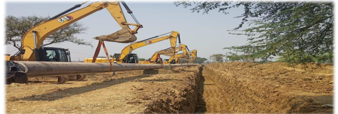
Setting up slurry pipeline
