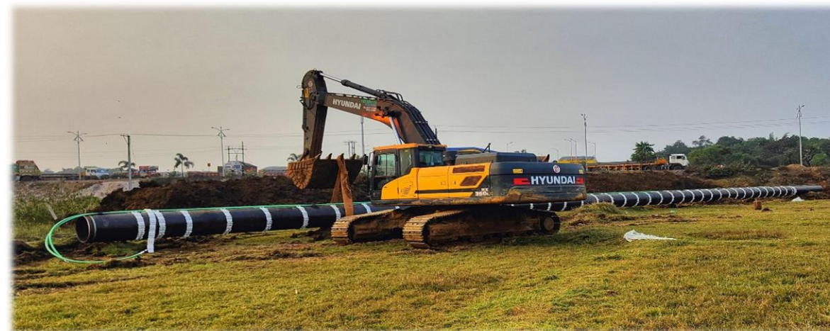
Setting up slurry pipeline
