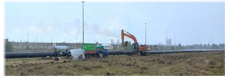
Setting up slurry pipeline
