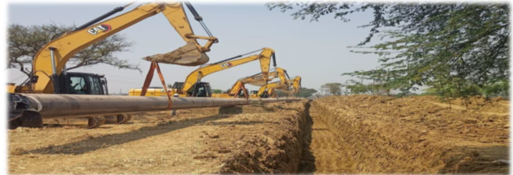
Setting up slurry pipeline
