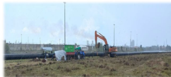
Setting up slurry pipeline
