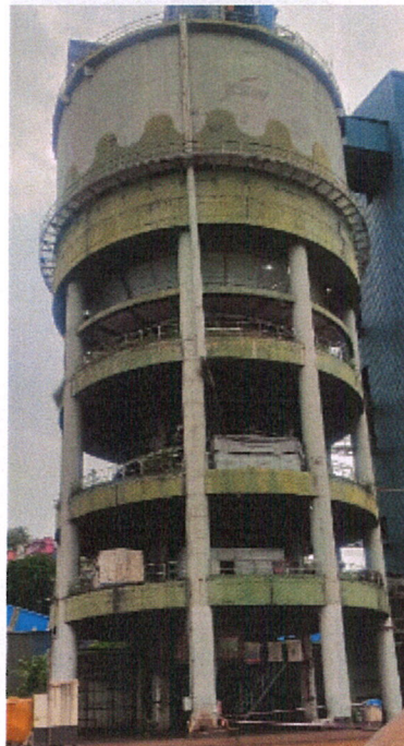
Silo loading attached with pipe conveyer
