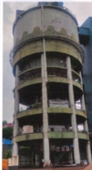
Silo loading attached with pipe conveyor
