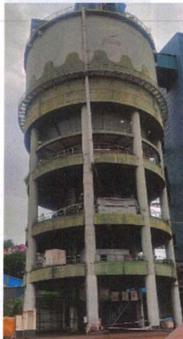
Silo loading attached with pipe conveyor
