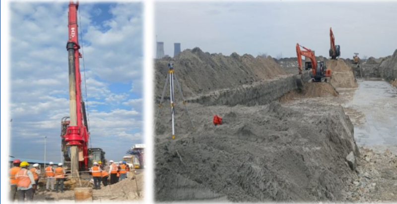
Images of Piling work and Stockyard at Tuticorin site
