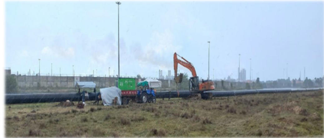
Setting up slurry pipeline
