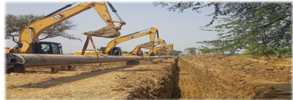
Setting up slurry pipeline
