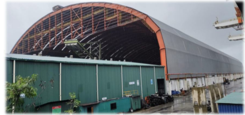
Cover shed work completed at South West Port, Goa
