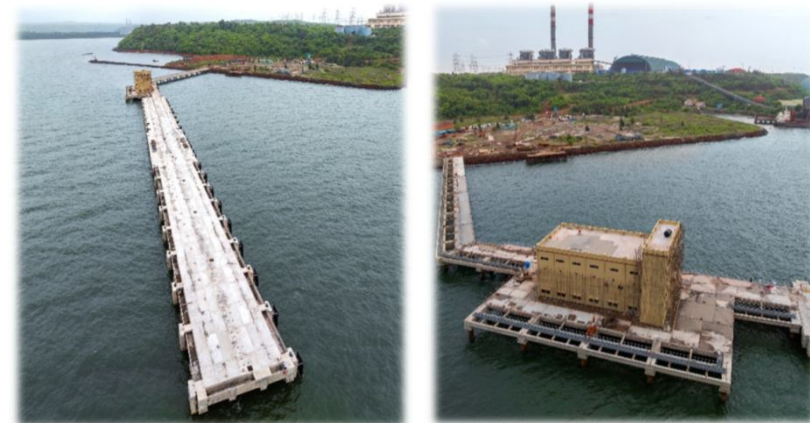
LPG construction at Jaigarh Port
